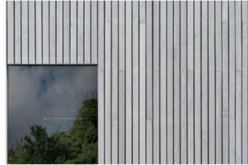
Timber Cladding to Upper Floor
