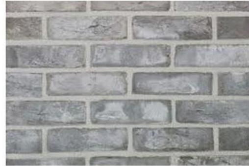
Facing Brickwork to Ground Floor
